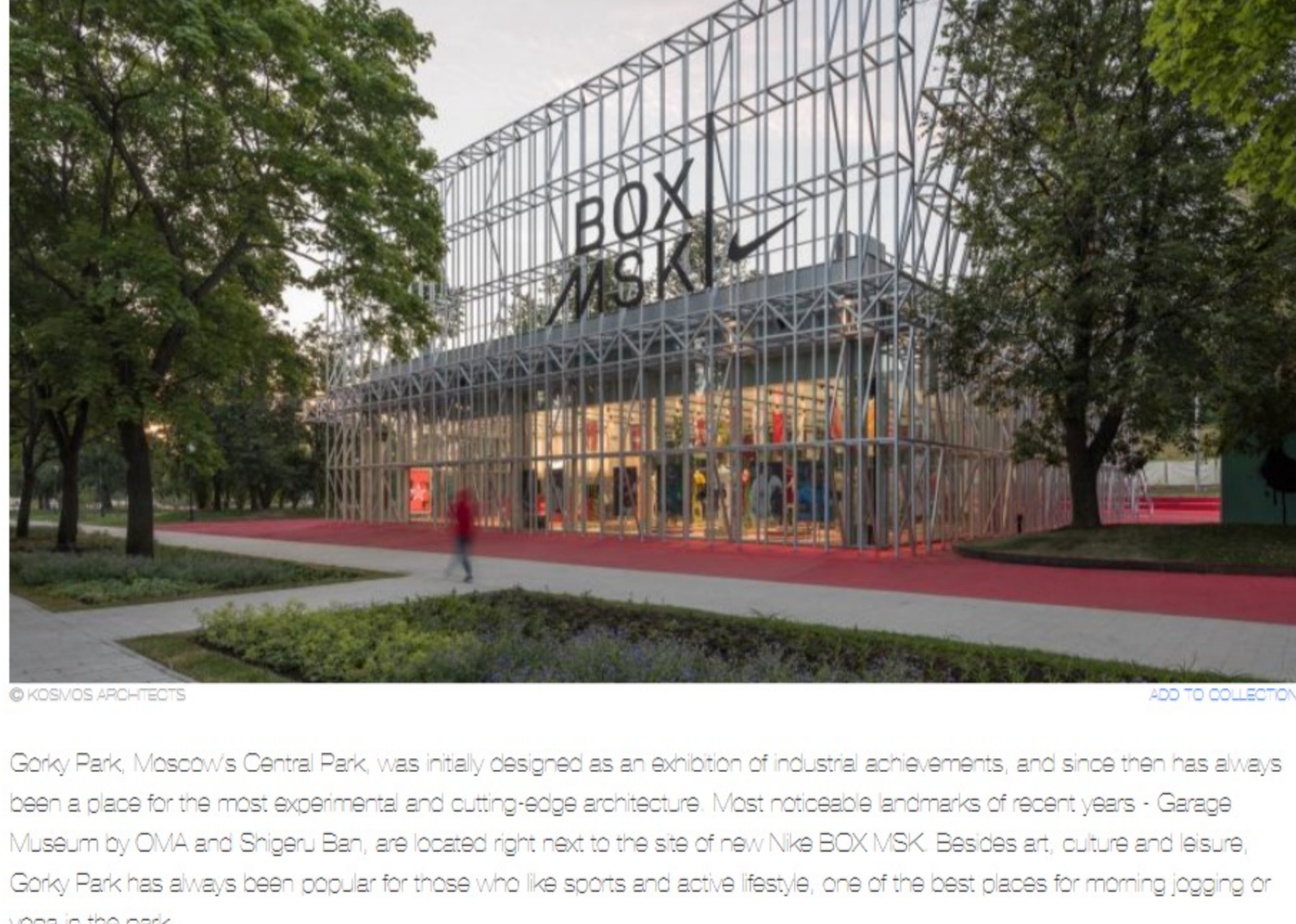
Gorky Park, Moscow's Central Park, was initially designed as an exhibition of industrial achievements, and since then has always been a place for the most experimental and cutting-edge architecture. Most noticeable examples of recent years - Garage Museum by OJIVA and Singur Bar, are located right next to the site of new Nike BOX M/SK. Besides art, culture and leisure, Gorky Park has always been popular for those who like sports and active lifestyle. One of the best places for morning jogging or yoga in the park.
